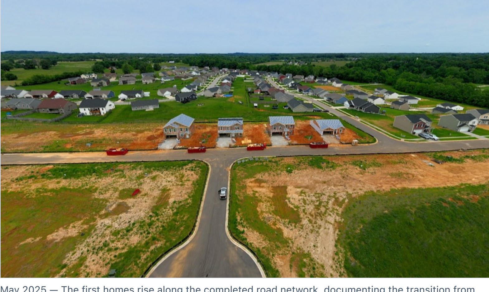
May 2025 — The first homes rise along the completed road network, documenting the transition from sitework to active building construction.
