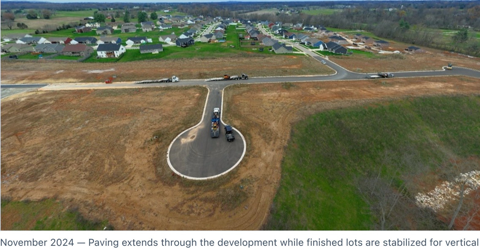
November 2024 — Paving extends through the development while finished lots are stabilized for vertical construction.
