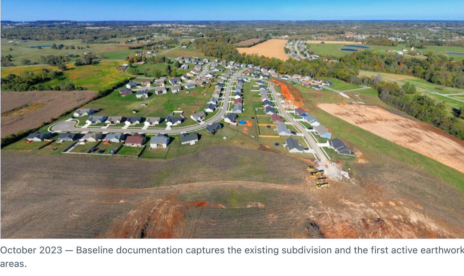
October 2023 — Baseline documentation captures the existing subdivision and the first active earthwork areas.
