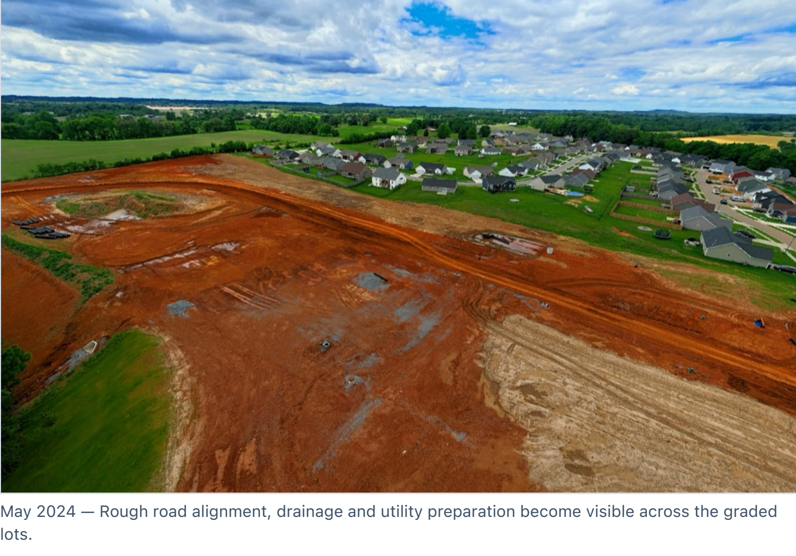
May 2024 — Rough road alignment, drainage and utility preparation become visible across the graded lots.
