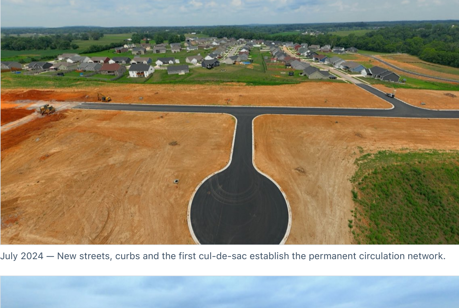
July 2024 — New streets, curbs and the first cul-de-sac establish the permanent circulation network.
