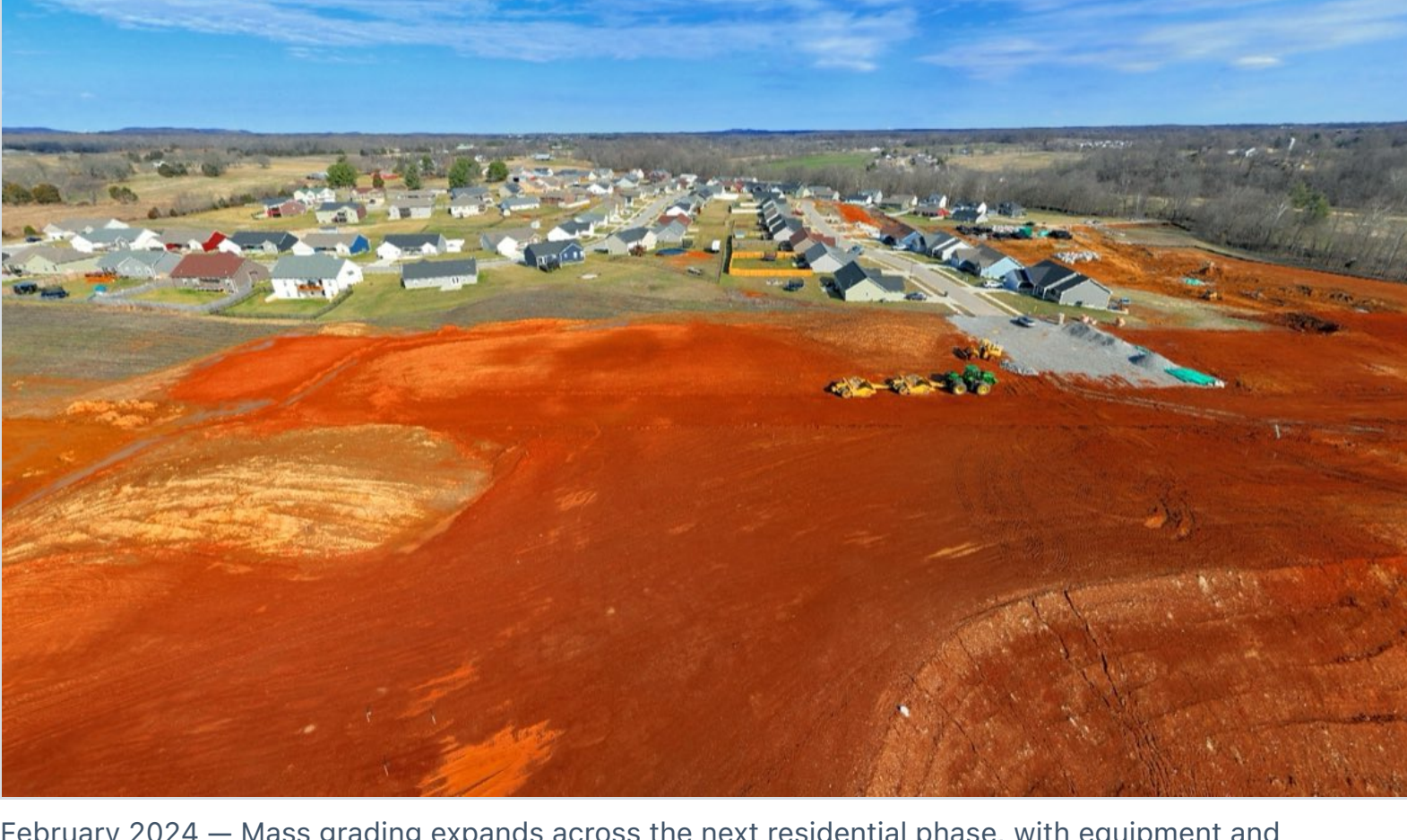
February 2024 — Mass grading expands across the next residential phase, with equipment and aggregate staged at the site entrance.
